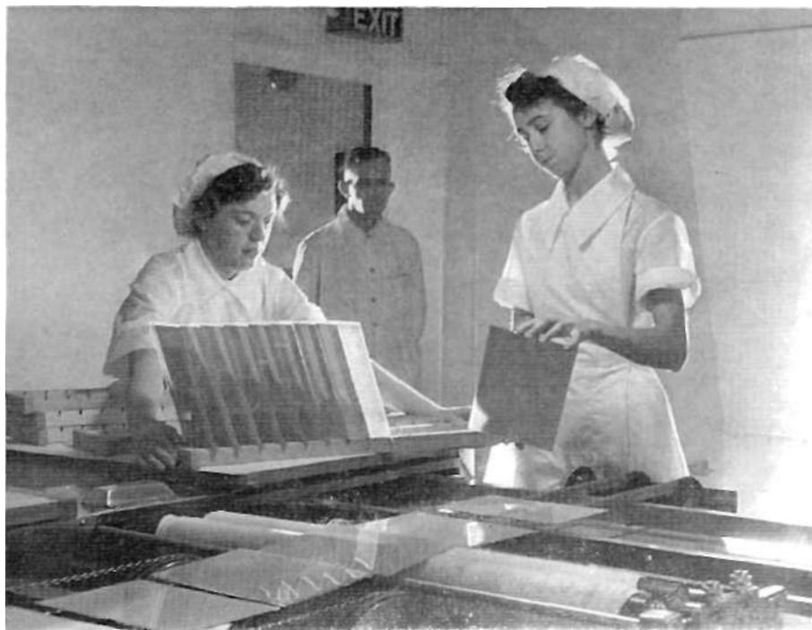
*Racking coated plates for drying.*
